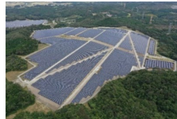
"Matsushima Donguri Solar Power Plant"
